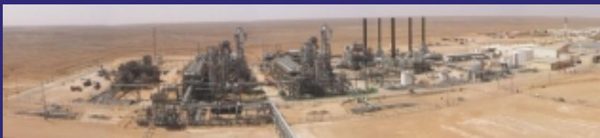
At this facility in Algeria, excess CO<sub>2</sub> is removed from natural gas for injection underground.
